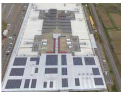
The roof of Kangawa Works after the installation of the photovoltaic generation system
